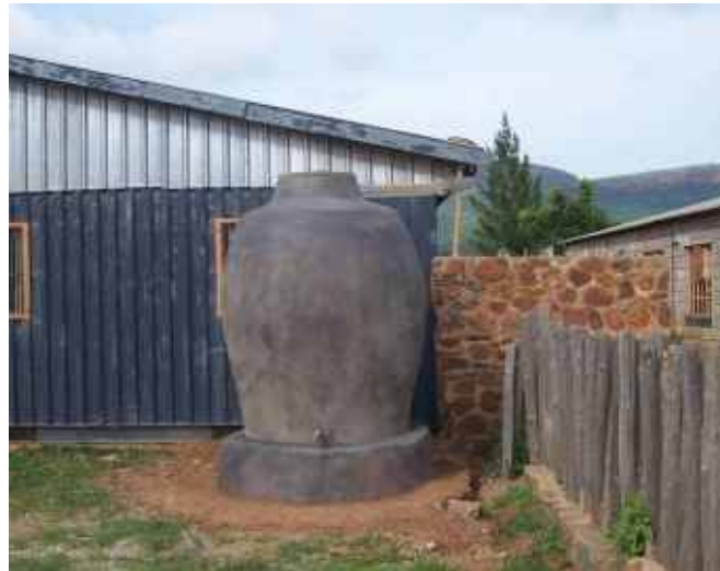
Rainwater harvesting tank built at the Kgautswane community centre.
