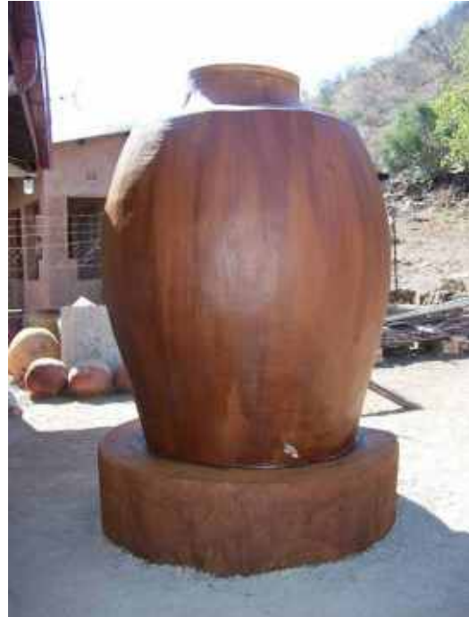
2,000 Litre Rainwater tank built on a pedestal.
